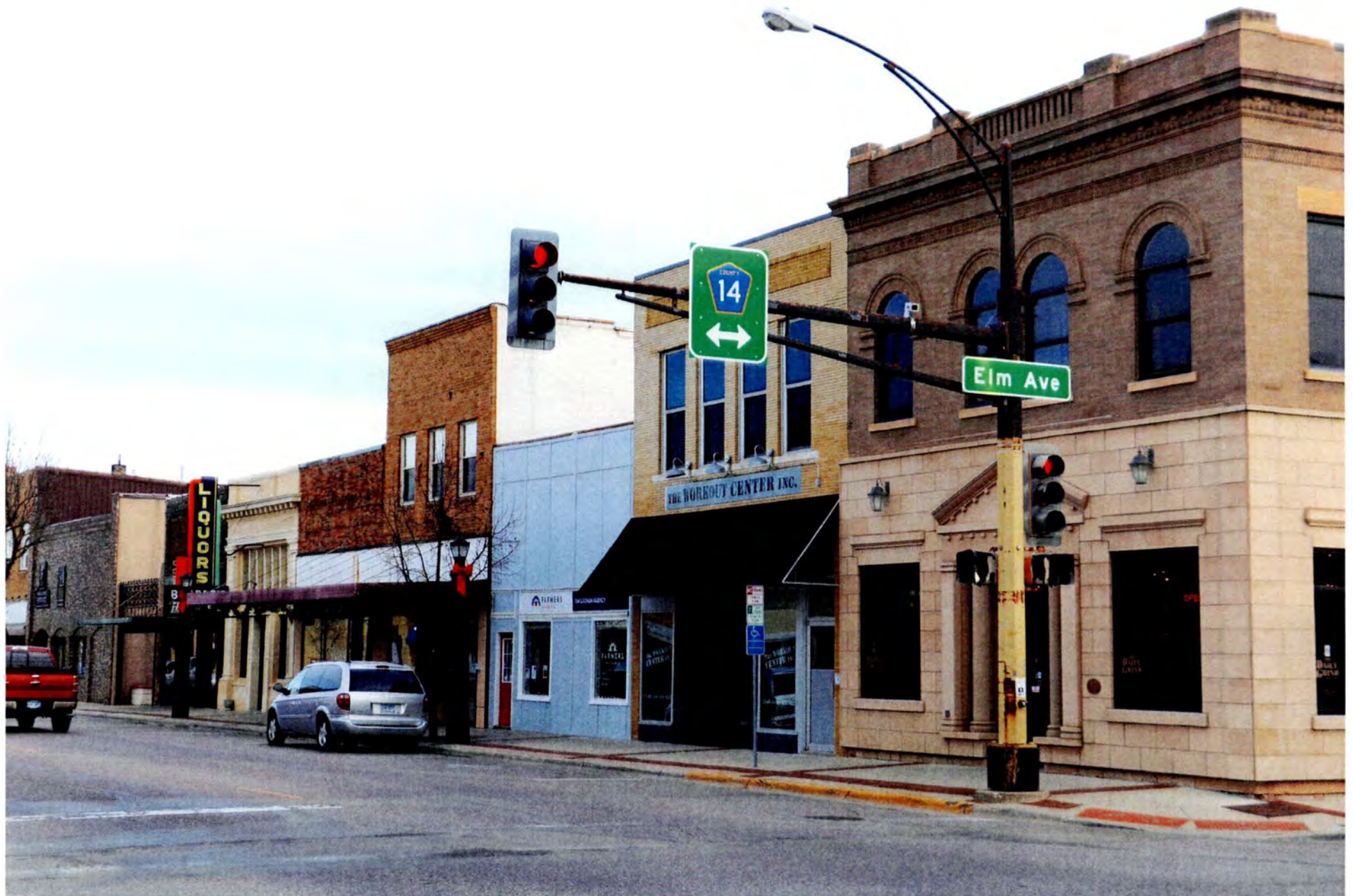
mn. waseca County - Waseca Commercial Historic District - 0005
