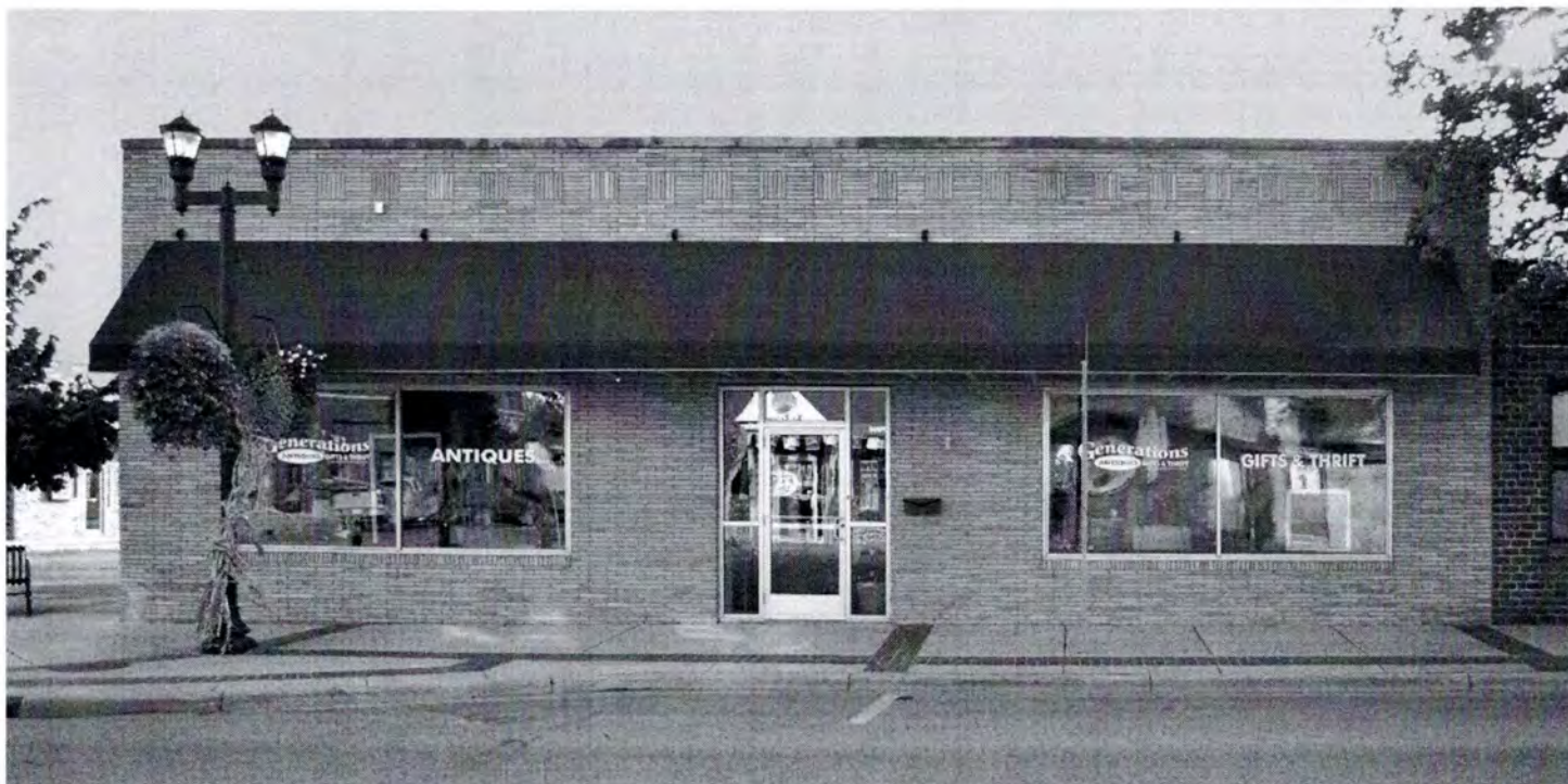
View looking east.
