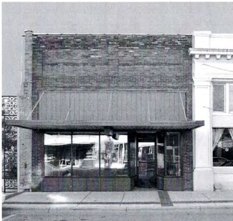
View looking east.
