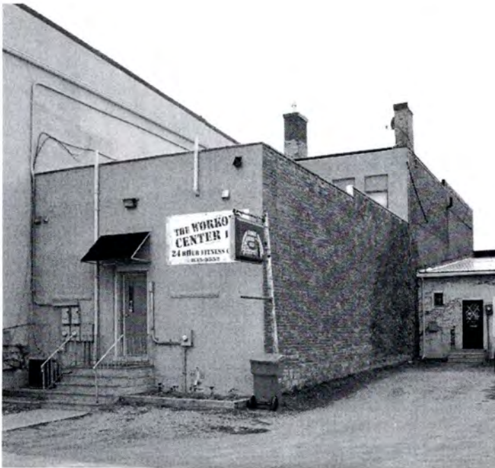
View looking southwest.
