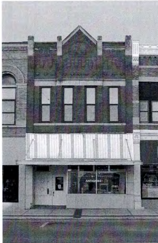
View looking east.
