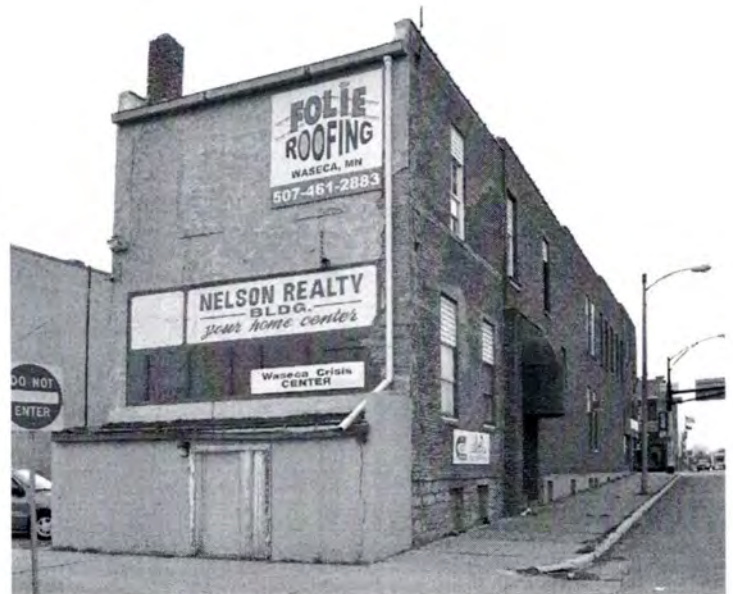
View looking southwest.
