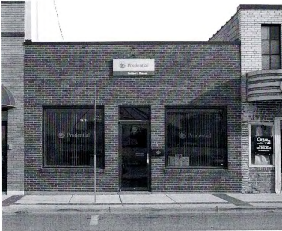
View looking east.
