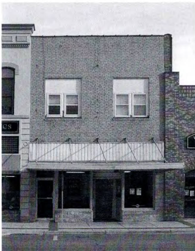
View looking east.
