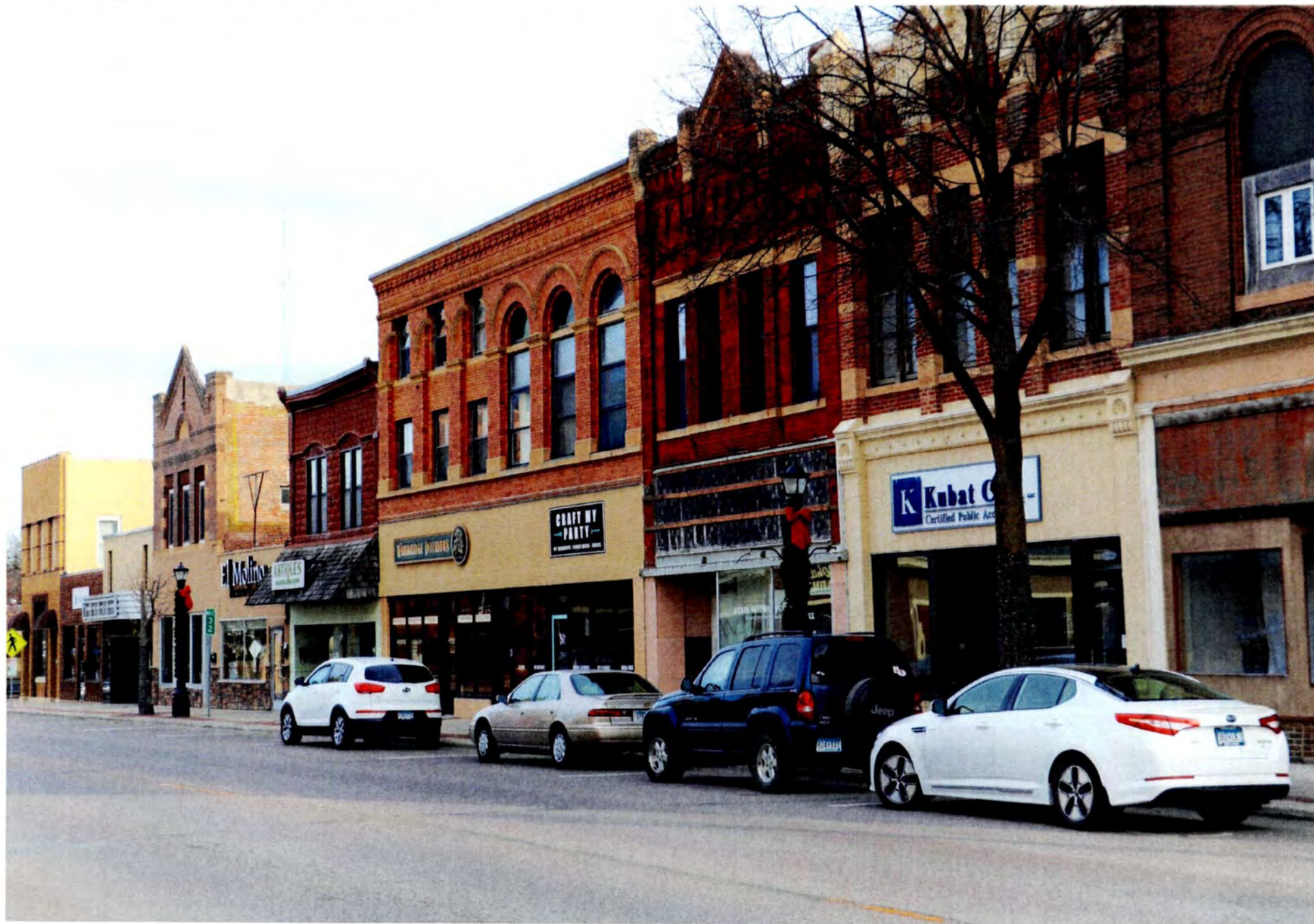
MN_Waseca County_Waseca Commercial Historic District_0008
